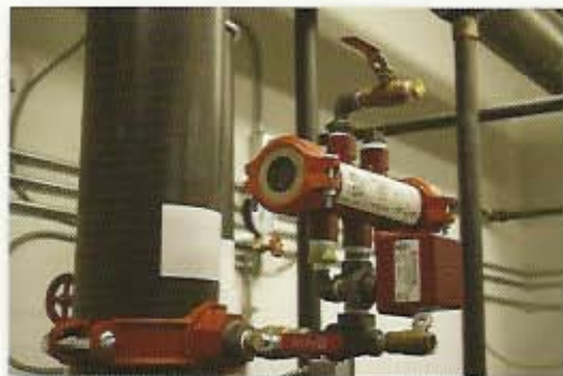
Potter Corrosion Monitoring Station Riser Mount
